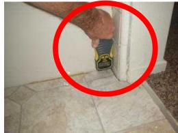
Acceptable, Safety Upgrade Shower/Surround: Gaps were noted which need to be sealed around the fixtures. Caulking all penetrations is highly recommended. Shower enclosure doors were not on the bottom track. Correction is recommended for added safety.
